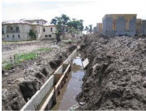
Wall construction continues.
